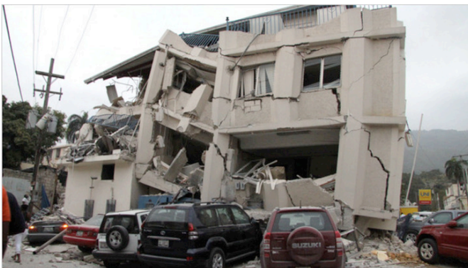
Earthquake in Haiti 2010
